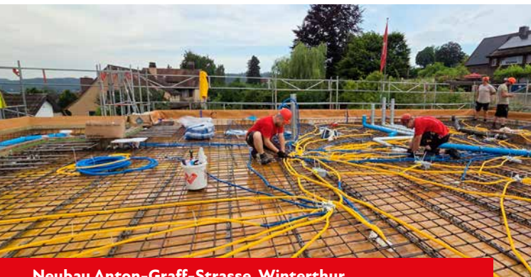
Neubau Anton-Graff-Strasse, Winterthur
